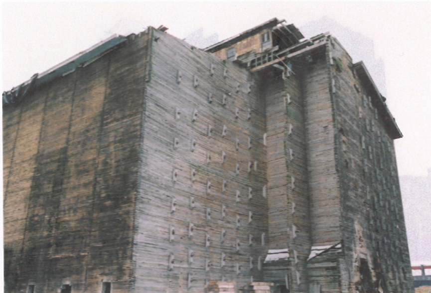
4 This elevator has been stripped of the corrugated iron that sheathed the wood, protecting the wheat, corn, and barley from the fierce winters of Lake Superior.
